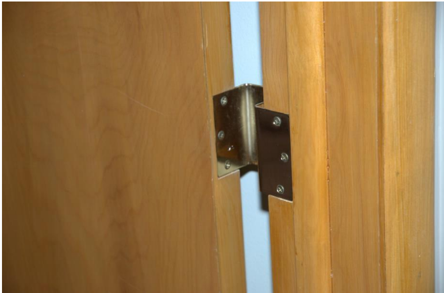
Adjust door hinges to create width.
