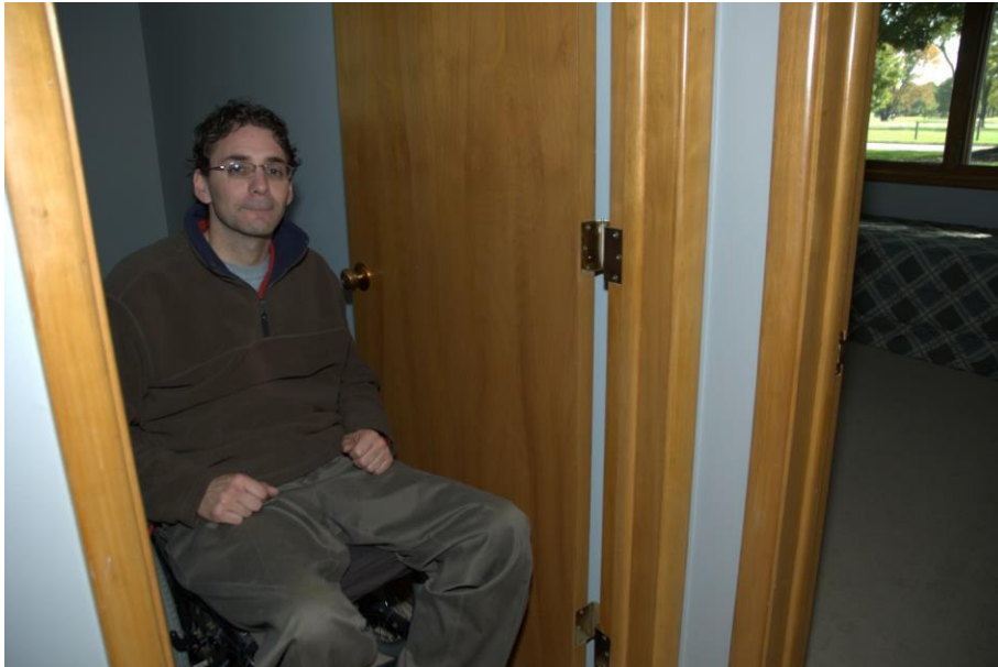
Door openings must be 32 inches wide to ensure a wheelchair can pass through.
